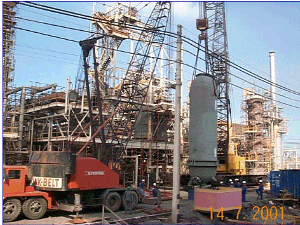
This photograph shows the Assembly of the New Converter
