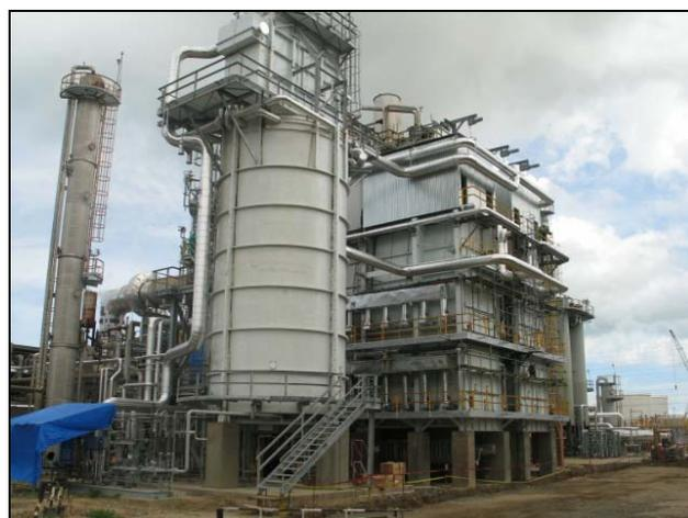
**Fig. 3 - Photo of the Primary Reformer and Fired Heater**
