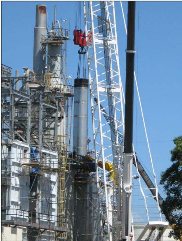
**Fig. 5 - Photo of Converter Basket being lifted into place**
