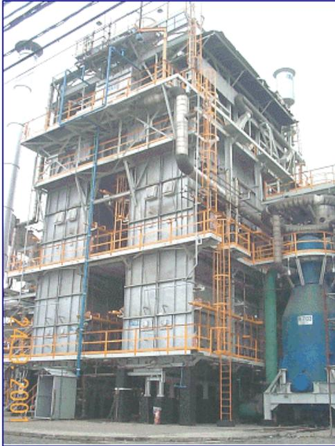
141,5 mm of external diameter and 9,5 mm thickness, which have an expected lifetime of 100.000 hrs. Before the revamp, the wall temperature was 950 °C (1742 °F) (Average) and after revamp, reduced down to 880 °C (1616 °F).
