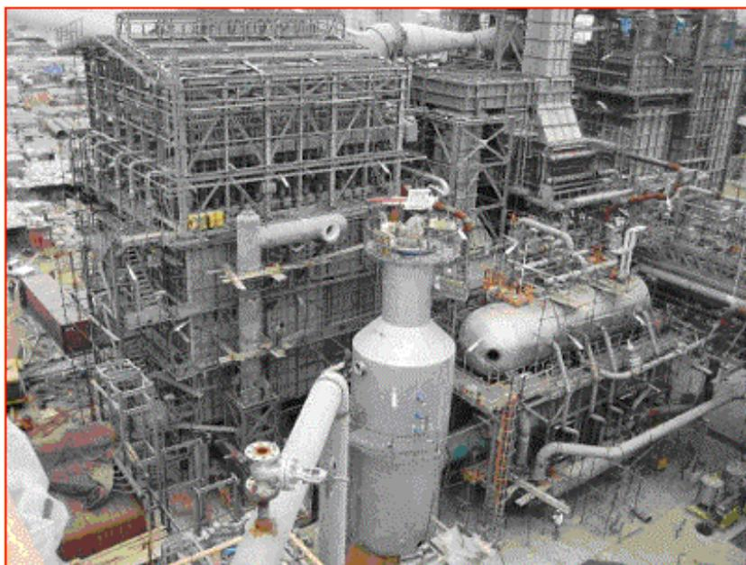
**Primary Reformer, Secondary Reformer Steam Drum & Waste Heat Boiler**
