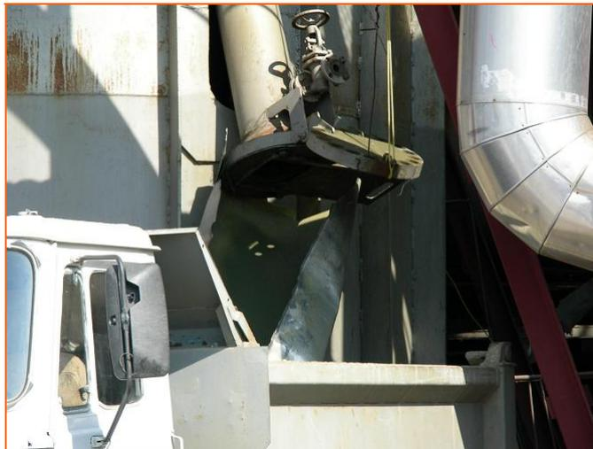
**Figure 10** – *Catalyst unloading in axial gas-cooled plate converter.*
