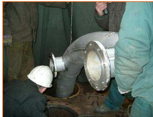
**Figure 8** – *"In situ" Installation of new internals.*
