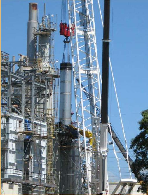
**Fig. 8 - Photo of the Converter Basket being lifted into place**
