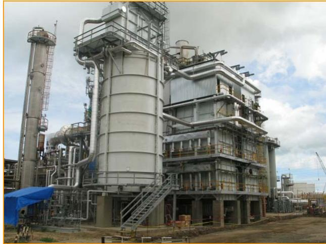
**Fig. 6 – Photo of the Primary Reformer and Fired Heater**
