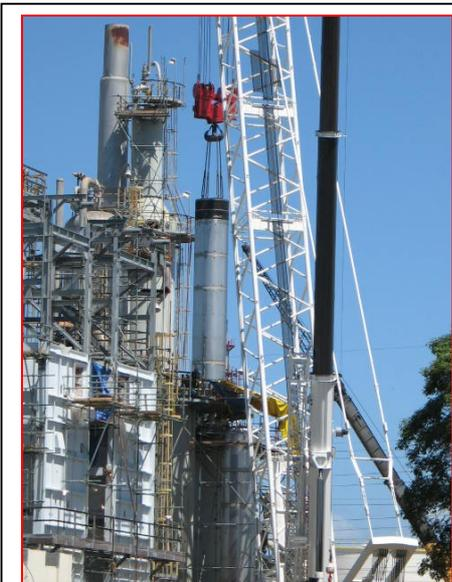
**Fig. 9 - Photo of IAC Converter Basket being lifted into place**
