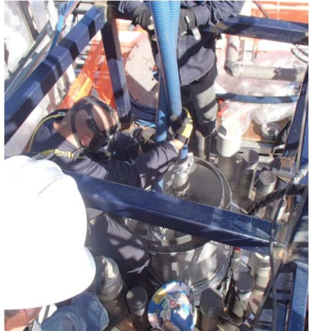
*Figure 9. Catalyst loading with hoses attached to special tool*
