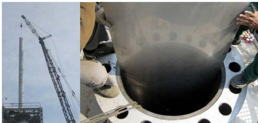
**Picture 2: Converter modules insertion in the vessel**
