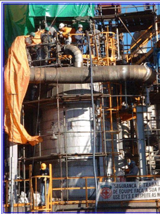
Figure 4 - Revamping of a POX HT shift converter in Brazil
