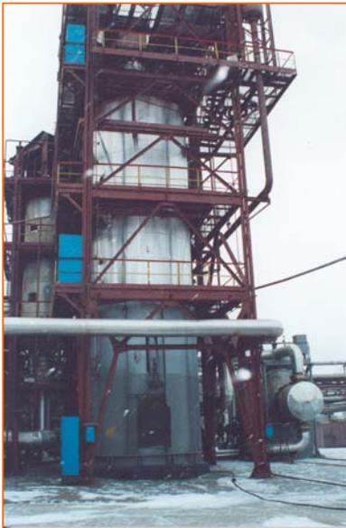
The plant where the converter internals have been installed is in Russia. Its old converter design was with adiabatic beds and quench cooling. The feedstock is acetylene off-gas enriched with hydrogen coming from an ammonia plant.
