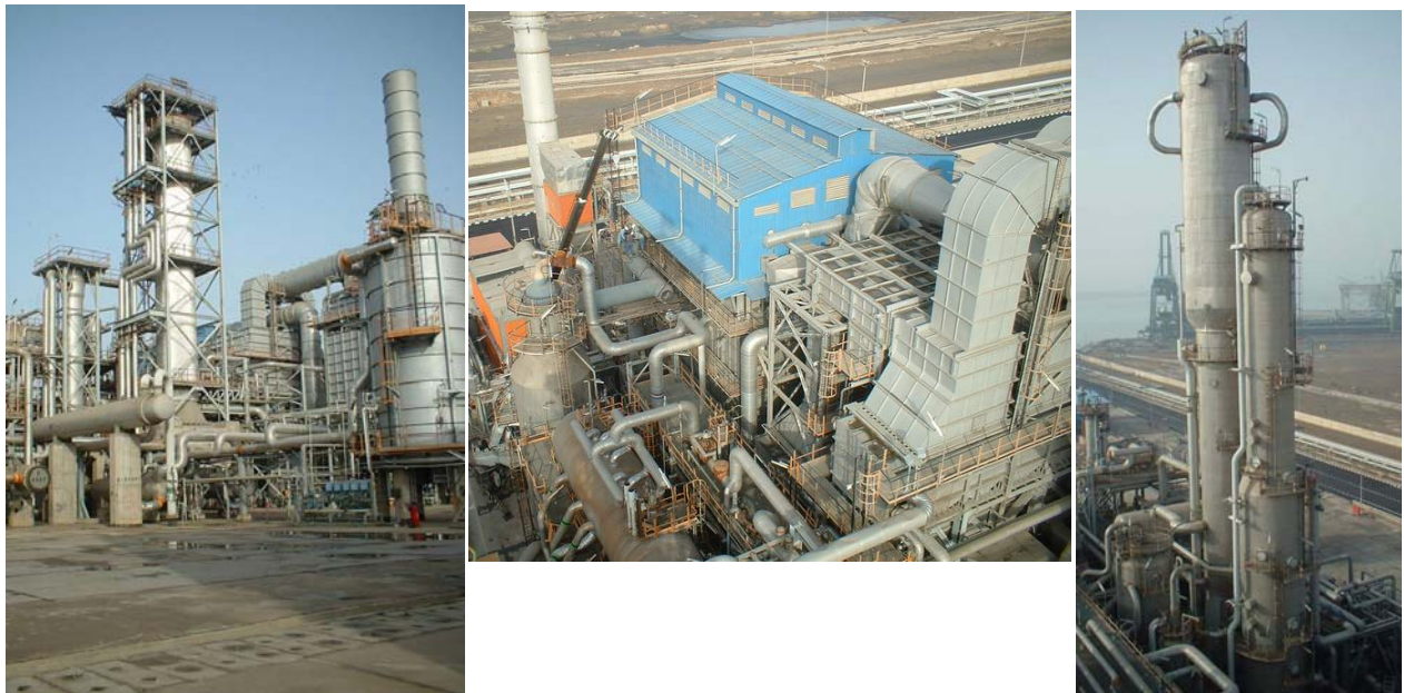
Fig. 14 - Casale Standard Ammonia process in operation in Iran
