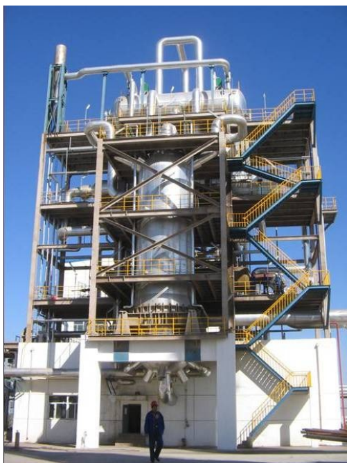
Figure 7. Picture of converter structure with steam drum on top level and DCS of Xinneng Energy Limited - Xin'ao Group plant
