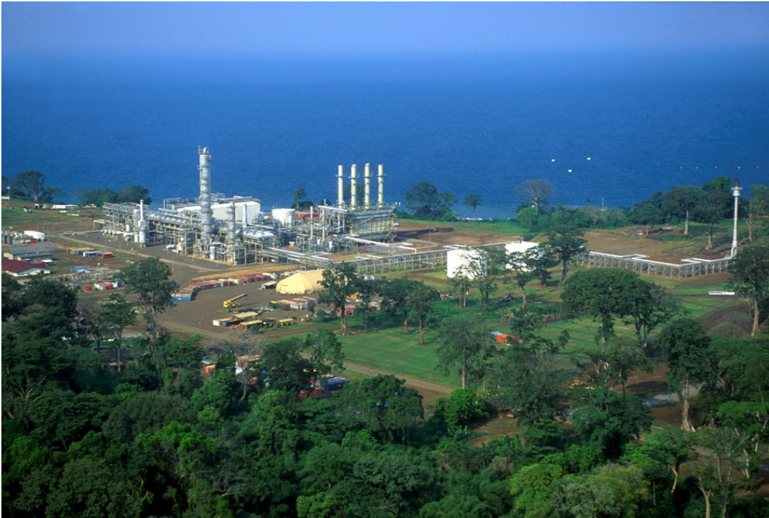
Overview of AMPCO production site
